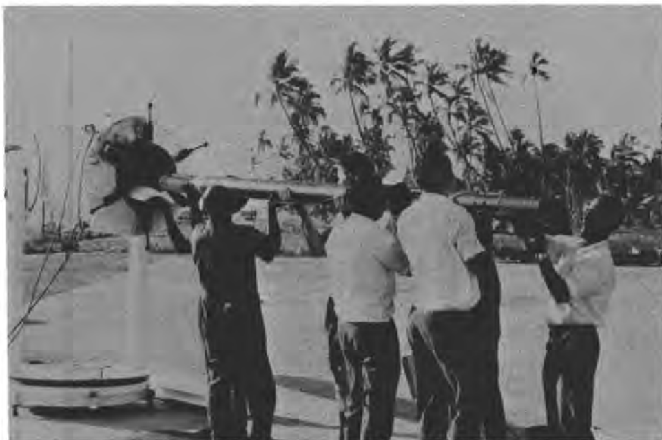
Arcas being loaded into launch tube, Thumba, India.
