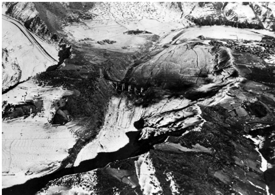
'Carlson's Canyon', the railway bridge and tunnel complex south of Kilchu, that became a battle of wits between naval aviators and North Korean engineers in March and April 1951. This image is dated March 2, 1951, before much damage had been done, and the supports for the unfinished parallel bridge are visible on the near side of the rail bridge. (US National Archive)
