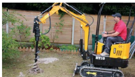
Drill for concrete piles
