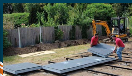
Lay steel subframe & floor panels
