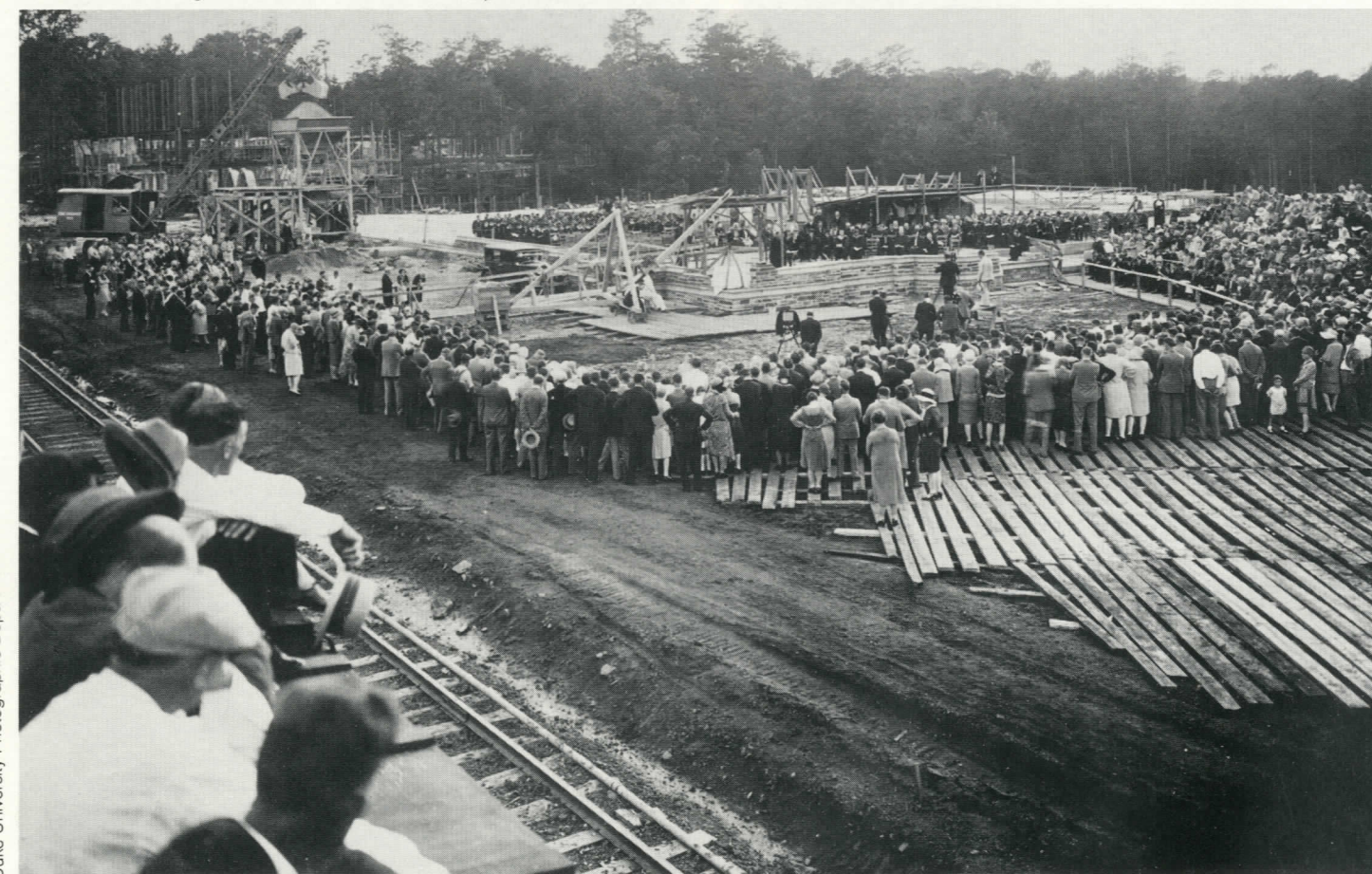
Laying the cornerstone of Duke's West Campus Union building, 5 June 1928.
