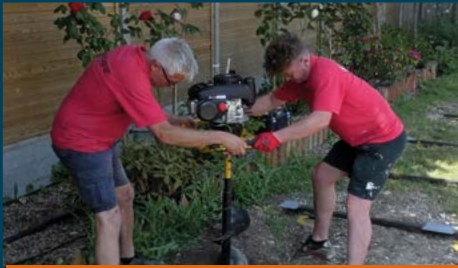
Drill for concrete piles
