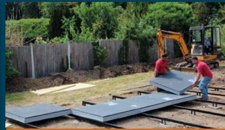
Lay steel subframe & floor panels
