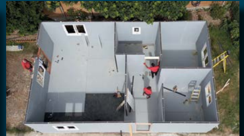
Erect wall panels & construct roof
