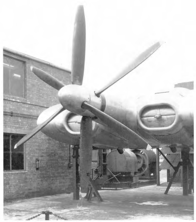
Above left: Although it turned out to be a failure, innovative engineering went into the Brabazon's design. This overhead view shows how each pair of Bristol Centaurus 20s was mounted. (Photo courtesy of the Bristol Branch of the Rolls-Royce Heritage Trust) Above right: In order to test out the Brabazon's unique powertrain, a wing section was made for this purpose. Convair did the same thing when developing the engine installation for the B-36. It's quite possible that Convair and Bristol engineers shared experiences developing their respective giants. (Photo courtesy of the Bristol Branch of the Rolls-Royce Heritage Trust)
