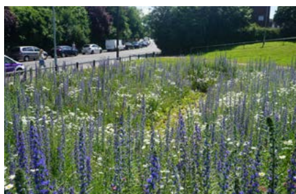
Bioswale part of SuDS for Severn Trent Water in Mansfield
