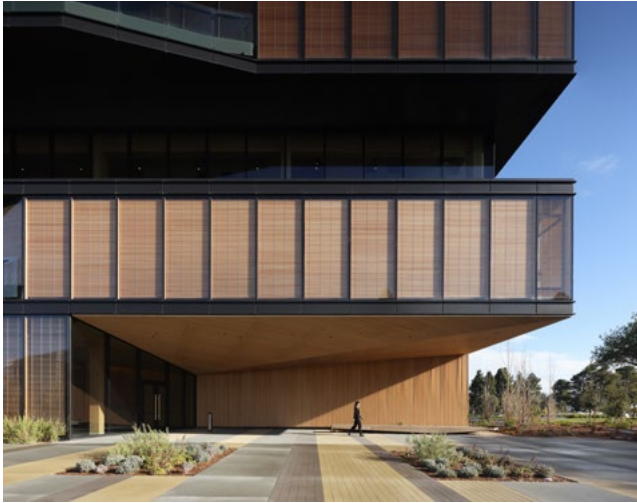
Google by MGA | Michael Green Architecture (Finalist, Best Large Firm) Photo: Ema Peter
