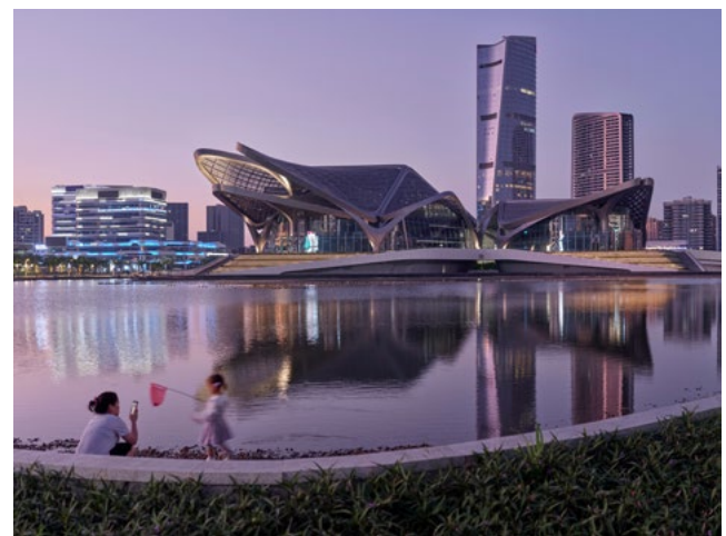
Zhuhai Jinwan Civic Art Centre by Zaha Hadid Architects (Finalist, Cultural & Expo Centers) Photo: Virgile Simon Bertrand
