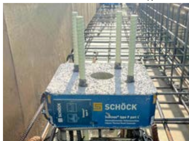
Sconnex type P on-site
