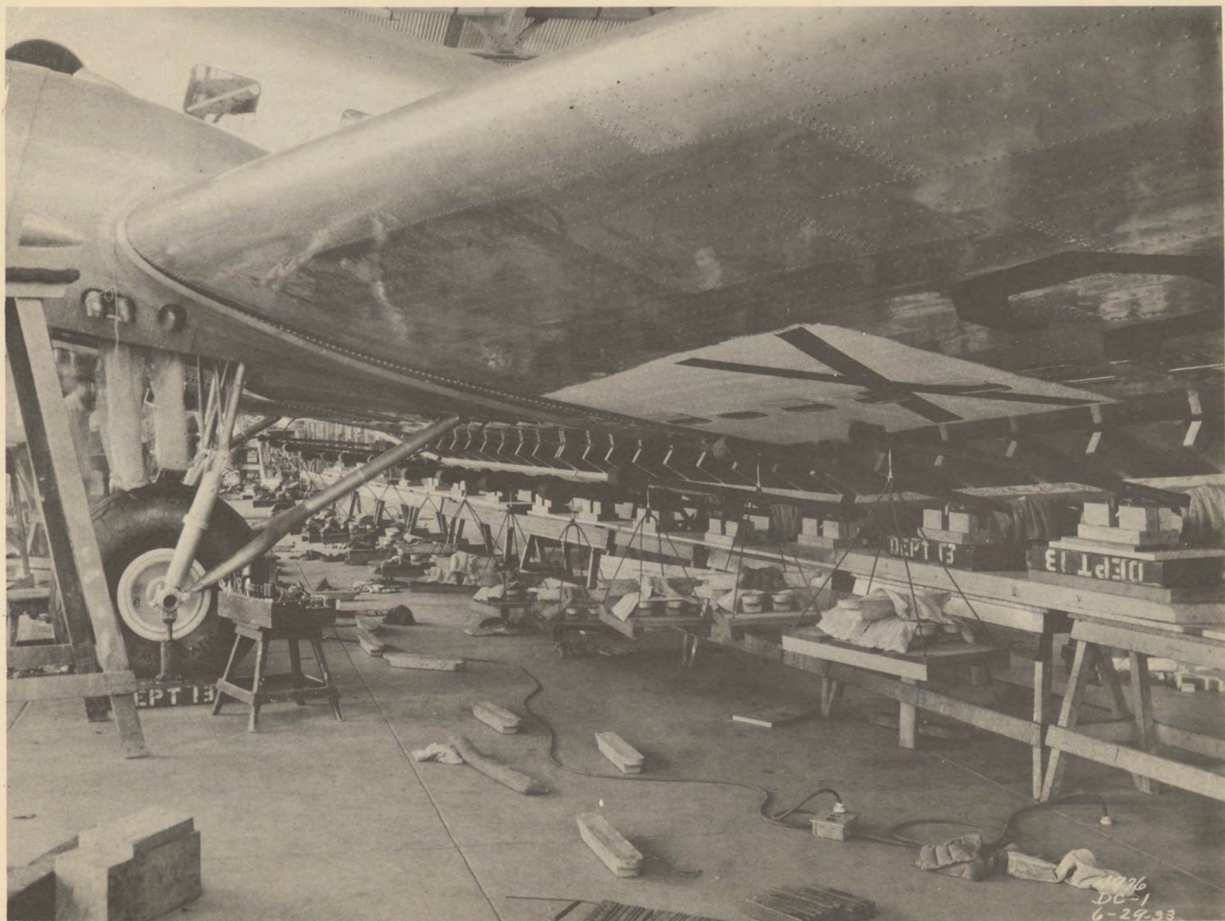
14996 DC-1 6-29-33 STATIC TEST OF WING FLAP AND CONTROL MECHANISM. (NOTE ACCESSIBILITY OF ENGINE NACELLE INTERIOR).
