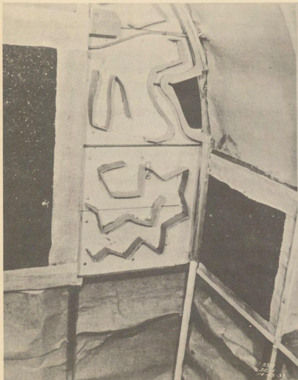
VARIOUS STAGES OF THE SOUNDPROOFING INSTALLATION IN THE FORWARD CABIN WALL.
