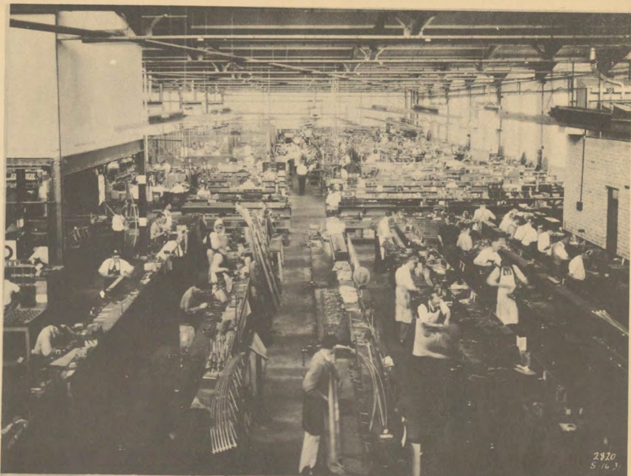
VIEW OF THE METAL FITTINGS DEPARTMENT AT THE DOUGLAS FACTORY THE SCREENED SECTION IN THE LEFT BACKGROUND IS AN INSPECTION BOOTH.
