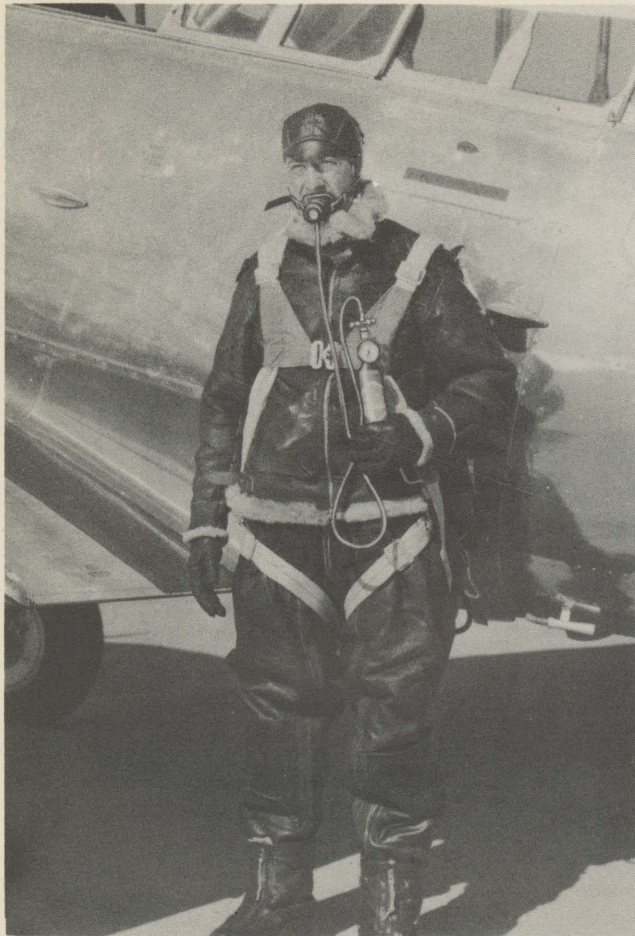
FIG. 22—BAIL-OUT CYLINDER UNIT
