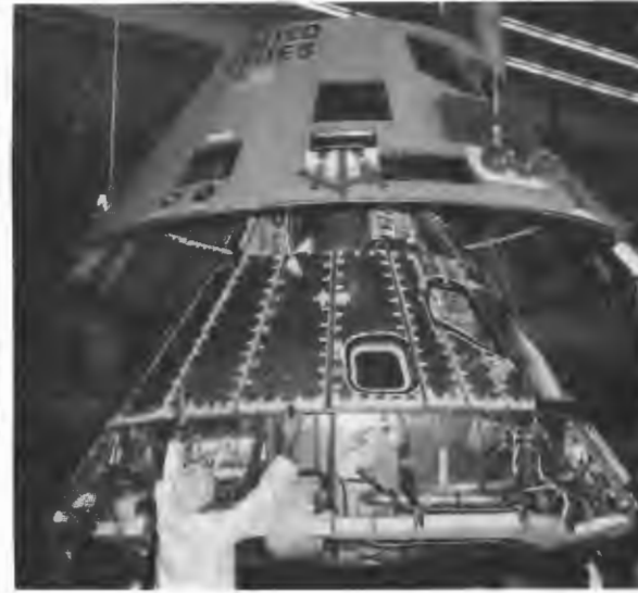
The drawing outlines major parts of the command module structure. In the photo at top right, the cabin section (or primary structure) of the CM is assembled at North American in 1965. Technicians (in the center left photo) work on the central heatshield, the two men on the sides applying heat-protection ablative material with caulking guns. A completed central heatshield in the bottom right photo is lowered into place over the primary structure in May 1966. In the bottom left photo, technicians prepare aft heatshields to attach to model CMs. These shields were made of fiberglass for test vehicles that did not require heat protection; the finished versions were of the same materials as the central heatshield.
