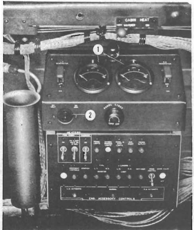
Figure 42A—Generator Control Panel (P-61B)
