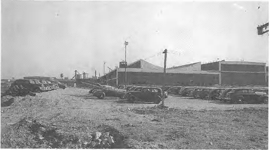
The two-story factory extension nears completion. This is on the north side of the complex. Photo courtesy of the Connecticut Air and Space Center, Stratford, CT.
