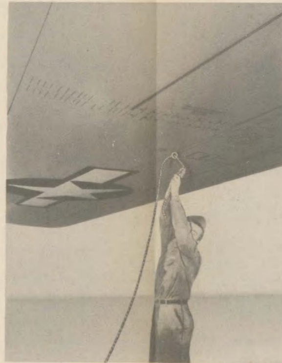
E ATTACHMENT TO WING EYEBOLT TIE DOWN FITTING
